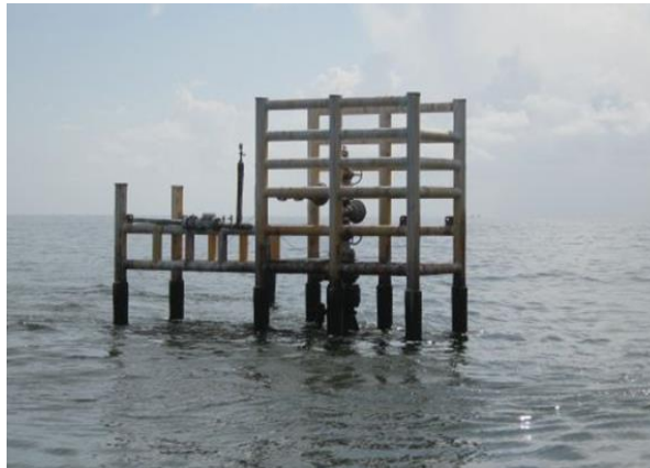
Suspended well with protection cage
