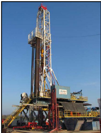
AD-1 Drilling Rig
