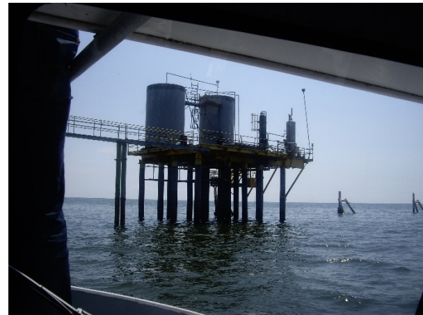
Storage tanks with walkway to facilities
