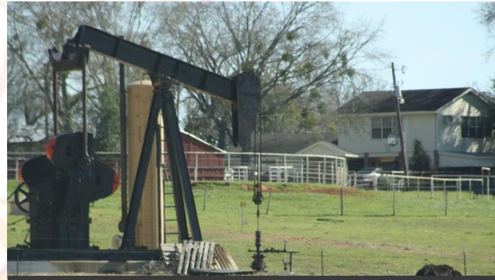
Existing vertical oil production
