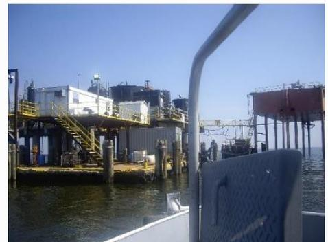
Figure 5: Example of an unmanned production facility which Sun Resources intends to utilise for development of Bowsprit. Source: Sun Resources
